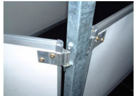
**Fig.1 Lifting the partition from the centre pole**
